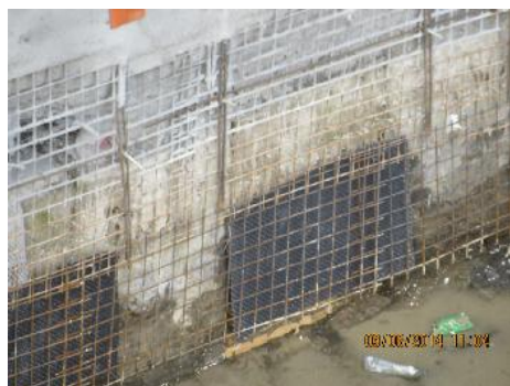
Figure 4: Implementation of horizontal drainage
