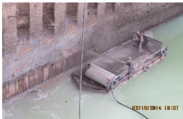
Figure 5: Implementation of Waterproofing concrete
