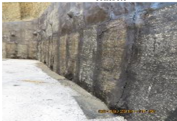
Figure 6: Implementation of impermeable 2-layer
