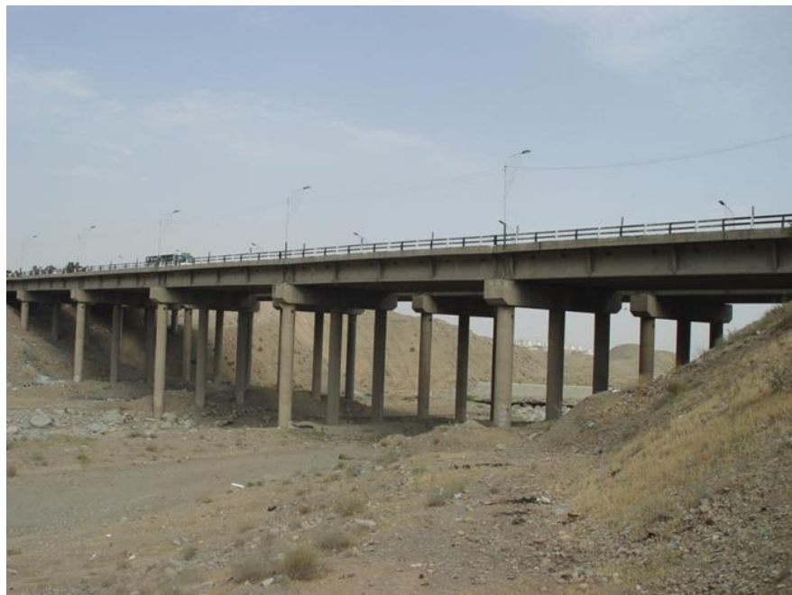
Figure 1: The view of studied bridge
