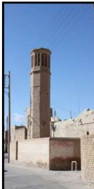
Figure 4: Ardestan's Sarhang-Abad Windcatcher
