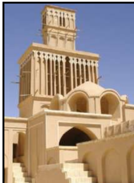
Figure 2: Two-Story Windcatcher of Aghazadeh of Abarkooh's House
