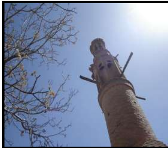
Figure 3: Polygonal Windcatcher of Nayin's Cistern (Source: Author)
