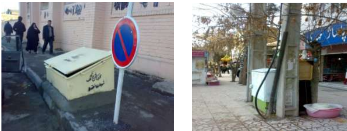
Figure 3: Inappropriate placing of city facilities on the sidewalks
