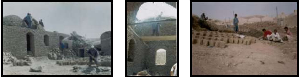
Figure 5: Process of making adobe, construction, and covering domed ceiling
