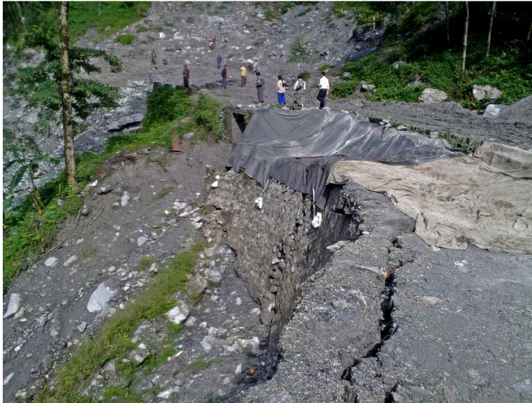
Figure 4: Gradual subsidence of the outer edge of the Hill Cart Road at Lower Paglajhora, 2010
