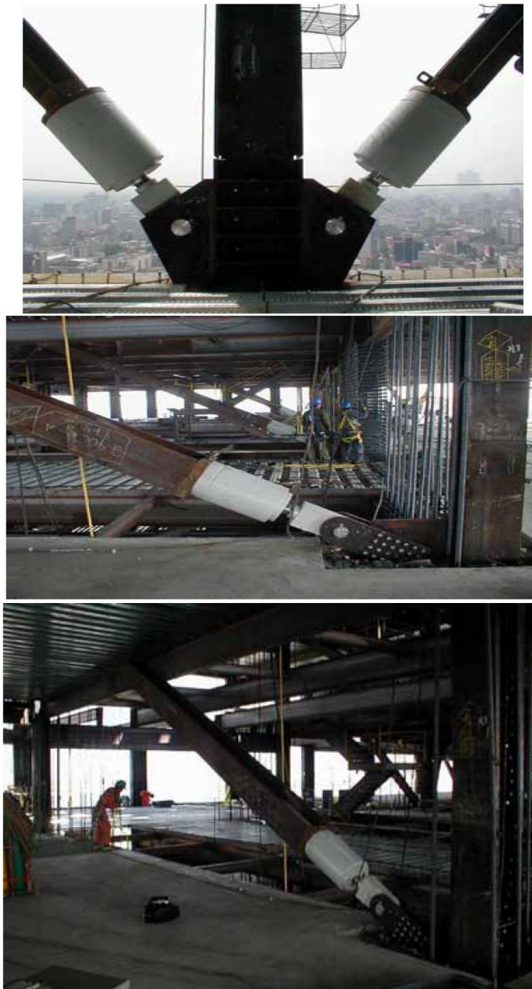
Figure 4: Application of dampers in the structure
