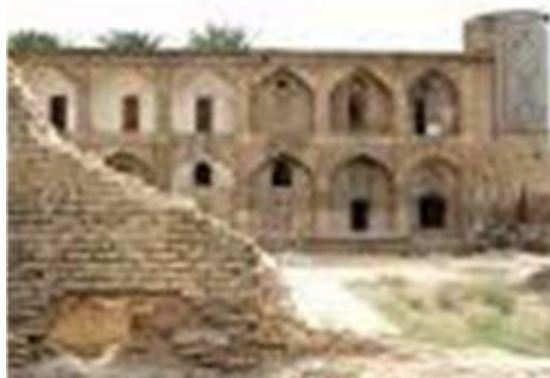
Image 5: The destructed chambers remained of the old fabric of Shiraz's Khan School
